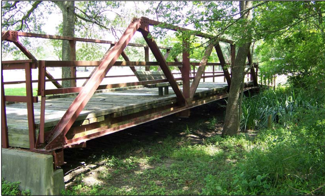
Figure 6. View of Warren Pony Truss Bridge
