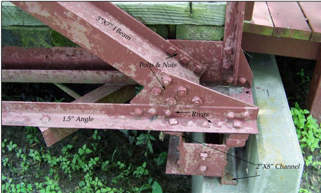
View of Corner Construction
