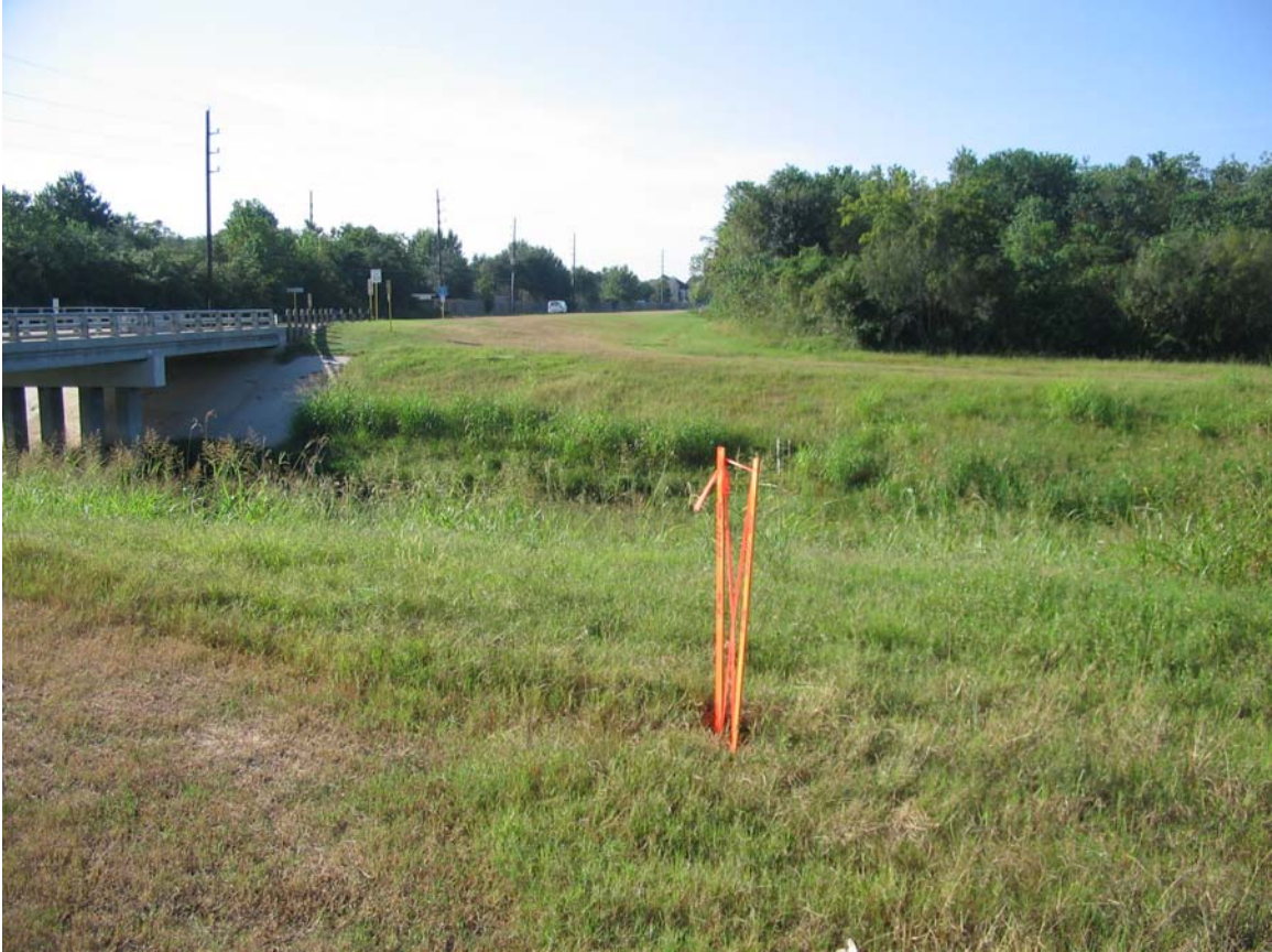
Figure 4. View of Channelized Bank of Dinner Creek
