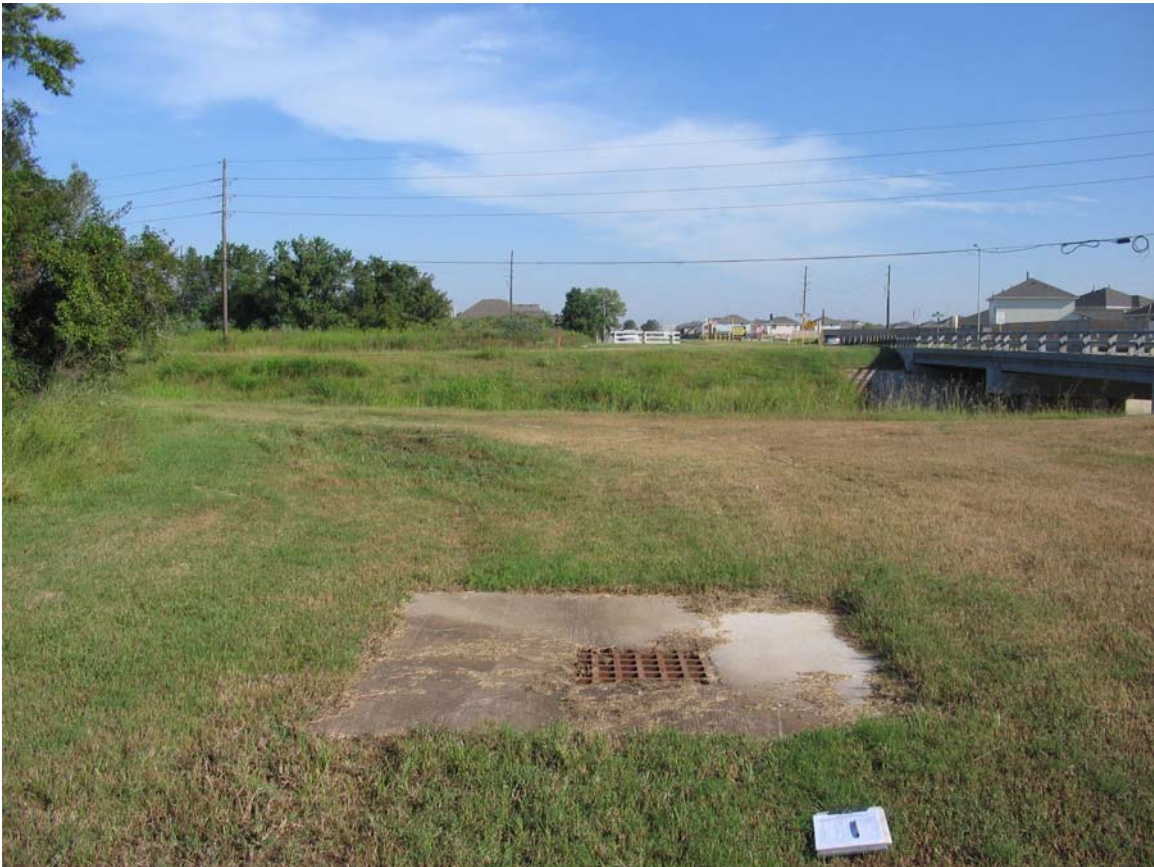
Figure 6. Storm Drain in Project Area
