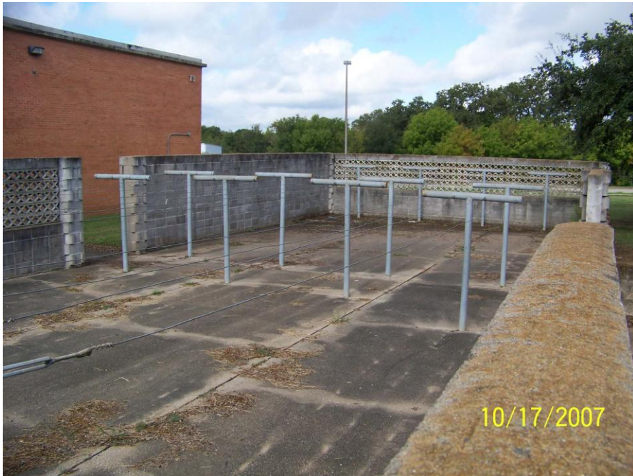
Building 531 – East Elevation (Clothesline)
