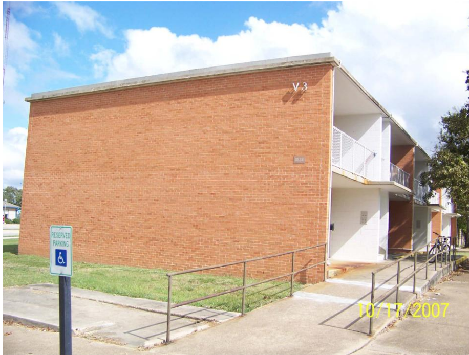
Building 534 – South/Southwest Elevation
