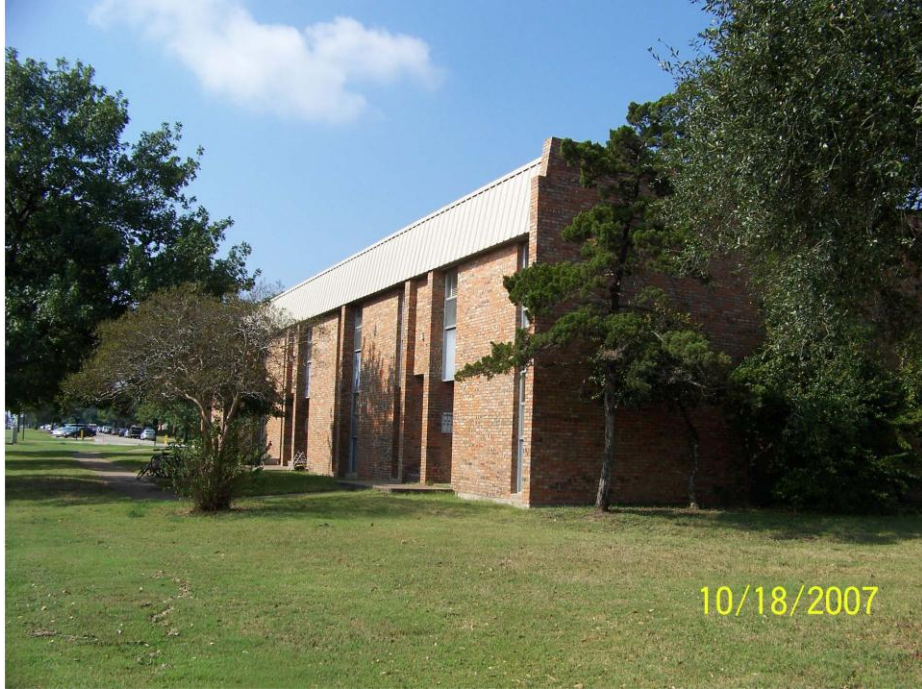
Building 1130 – Northeast Elevation
