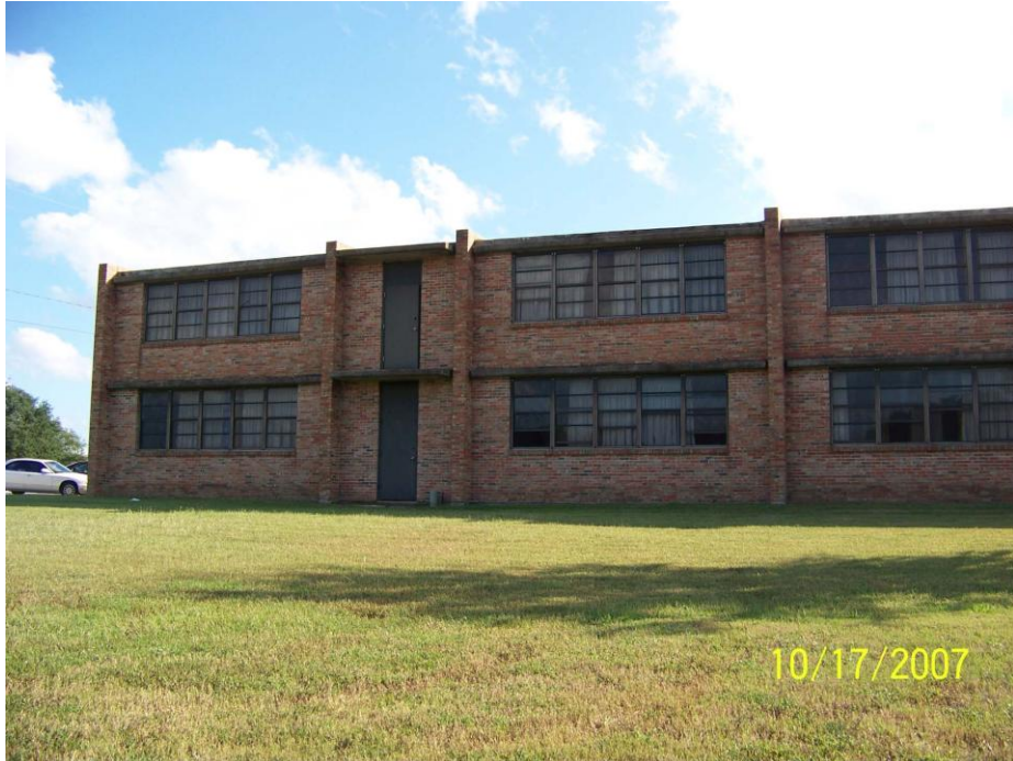
Building 1136 – Northwest Elevation
