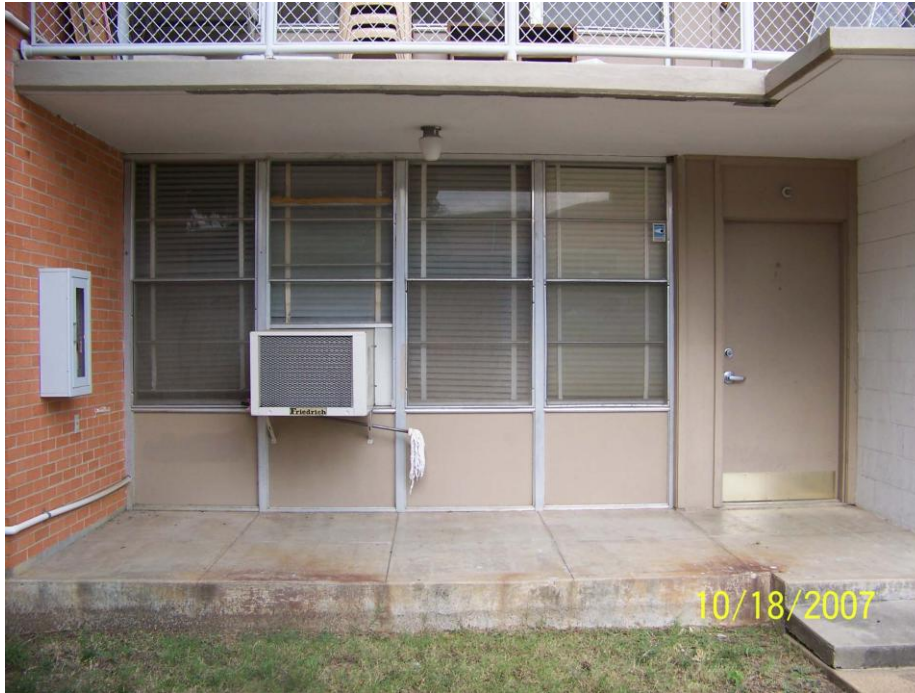
Building 529 – South Elevation (downstairs)
