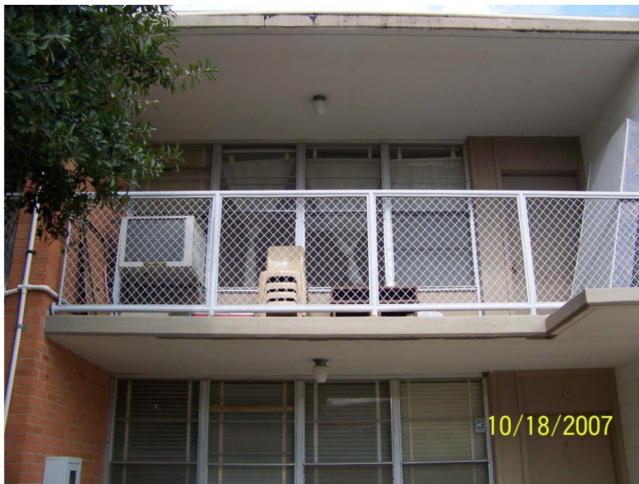
Building 529 – South Elevation (upstairs)
