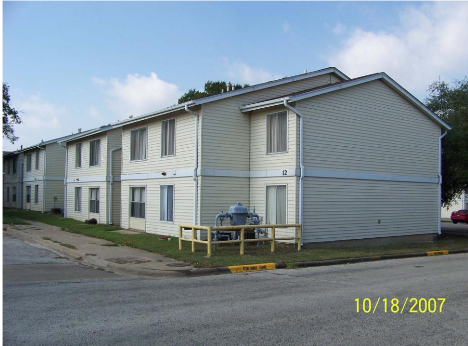
Building 1118 – Northeast Elevation
