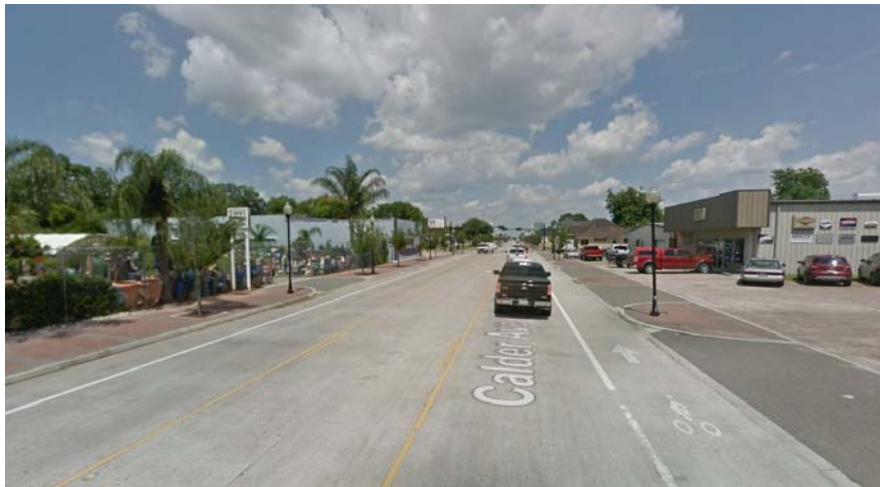
Figure 11: Street Segment with Existing Bicycle Lane, City of Beaumont, Jefferson County
