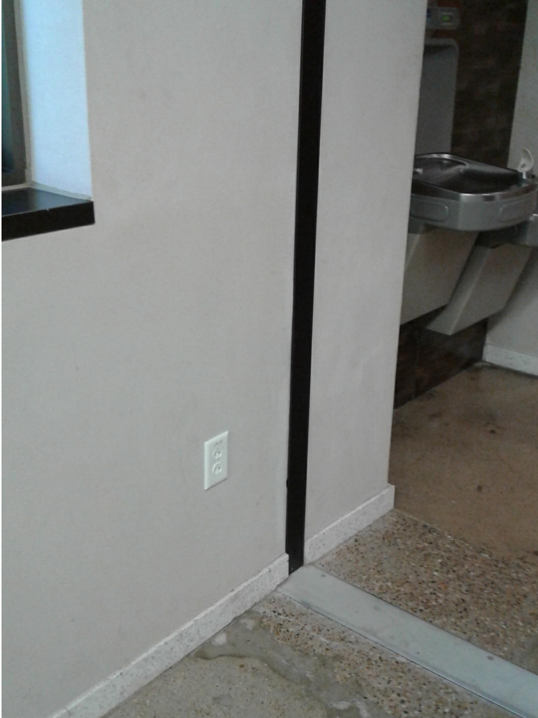
Figure 2. Building Expansion Joint between FH original and Addition
