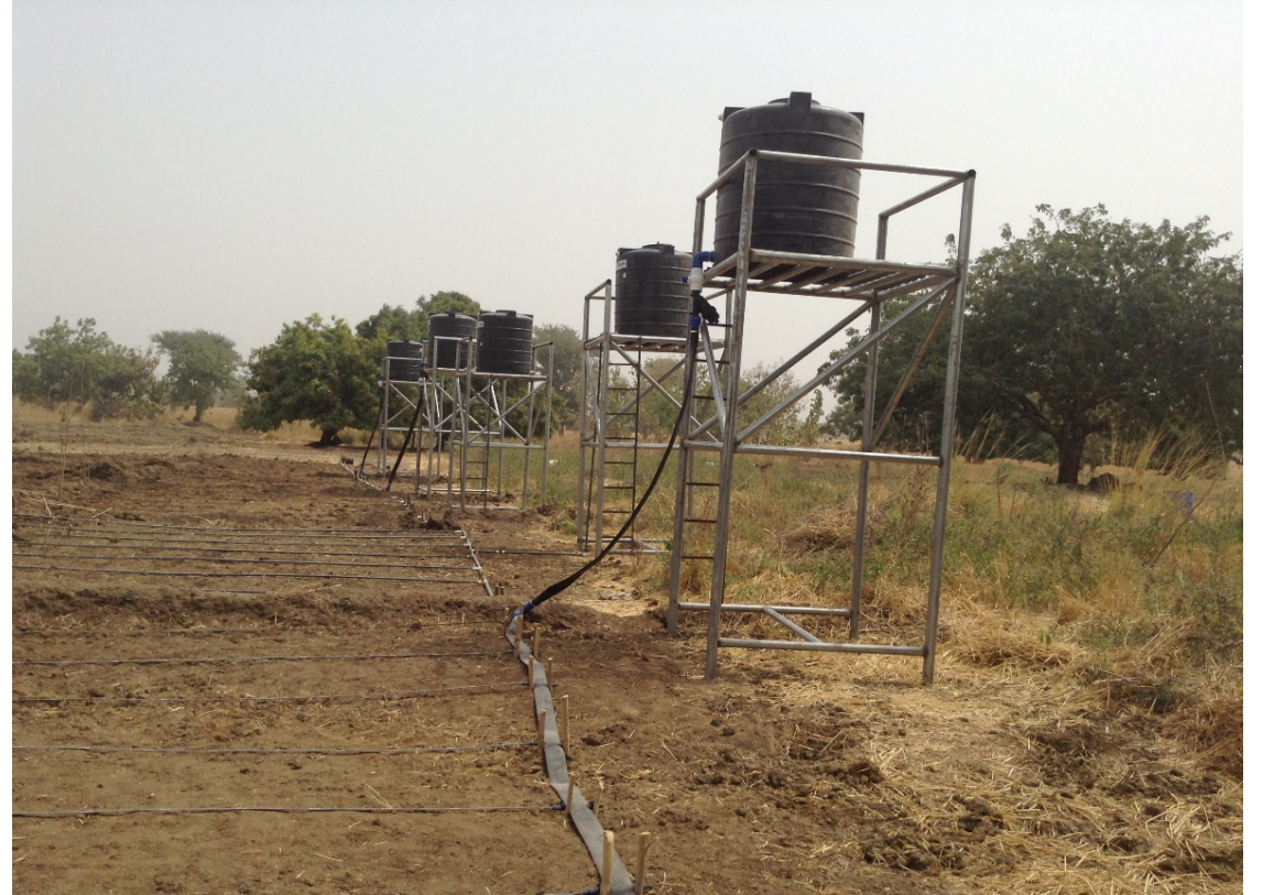
Water tanks installed at Dimbasinia
