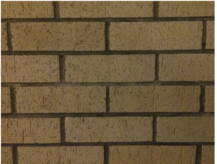
Figure 33. (below) typical masonry with slight coloration of mortar; field survey, November 30, 2017.
