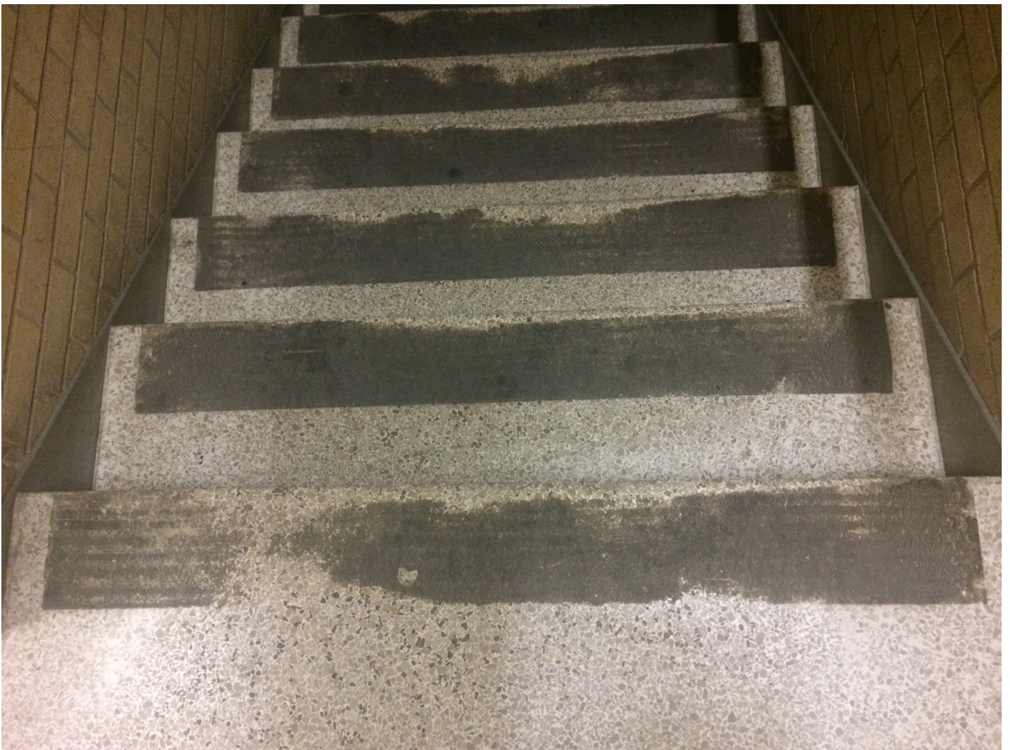
Figure 46. (below) West stairwell; field survey, November 30, 2017.
