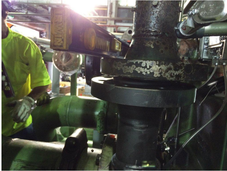
Figure 9: Piping Misalignment
