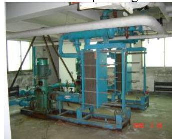
Fig.2 Photo of combined exchanger and equipped pump
